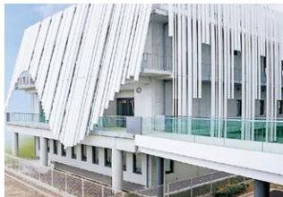
Integrated Research Center of Kobe University (Bio-Manufacturing Building)
